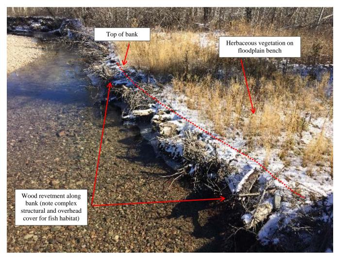
Figure 118. Wood revetment installed along river bank to prevent bank erosion, establish suitable channel width, and improve fish habitat (cover and refuge).
