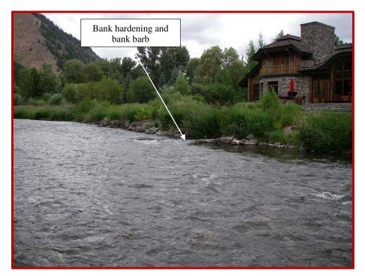
Figure 48. Photograph depicting bank stabilization and development encroachment in Ski Hill Reach.
