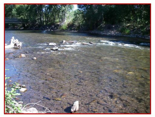
Figure 82. Photograph depicting typical channel confinement and failing rock sill structure in the Bullion Bridge Reach.
