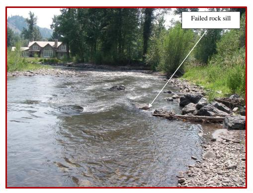
Figure 64. Photograph depicting failed rock sill and development encroachment in the Highway 75 Reach.
