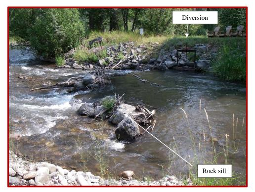
Figure 63. Photograph of river right diversion structure in the Highway 75 Reach.
