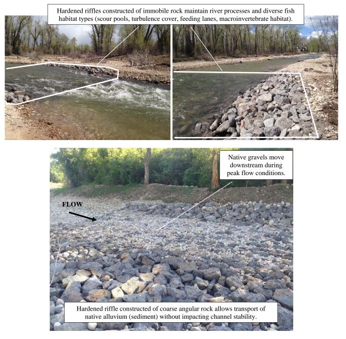
Figure 130. Hardened riffles maintain vertical channel stability and establish design channel width while maintaining downstream scour pools (top left and right). The hardened riffle treatment enables conveyance of native alluvium (sediment transport) while maintaining channel stability using moderately sized rock (bottom).
