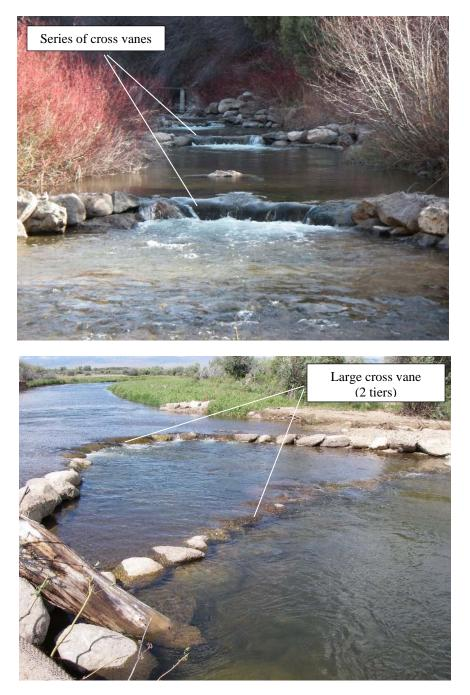
Figure 131. A series of rock cross vanes (top) distributes excessive local gradient while enabling sediment transport and maintaining downstream pools and mid-channel turbulence cover for fish habitat. A single large rock cross vane (bottom) maintains grade control and channel width while consolidating low flows in the center of the channel for hydraulic and fisheries benefits.
