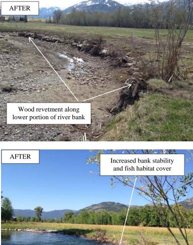
Figure 119. A severely eroding river bank (top) was stabilized with the wood revetment treatment (middle). The treatment effectively reduces potential for bank erosion, reduces near-bank flow velocities and erosive energy, and dramatically increases fish habitat through establishment of cover (structural, wood, and overhead).
