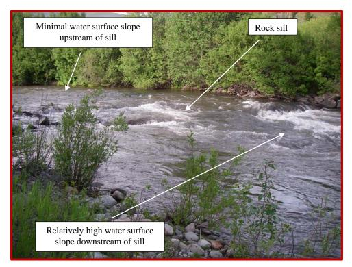
Figure 31. Photograph depicting an installed rock sill at near bankfull conditions in the Training Channel Reach.
