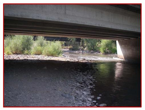
Figure 60. Photograph depicting sedimentation and point bar enlargement under highway bridge in the Highway 75 Reach.
