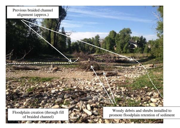
Figure 126. Photograph depicting created floodplain in a braided river system. An over-widened, dispersed, and braided river channel was filled to create floodplain and enable floodwater dispersal through the riparian area. Eroded areas were filled to create additional floodplain and re-establish a stable river channel to achieve sediment transport restoration and fish habitat enhancement objectives. The treatment enabled flood water dispersal, inundation, and groundwater recharge.
