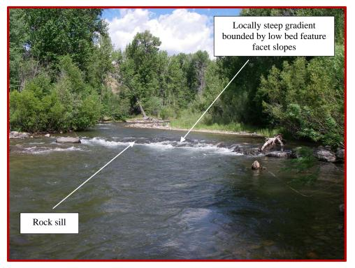
Figure 30. Photograph depicting an installed rock sill and localized confinement of available gradient in the Training Channel Reach.
