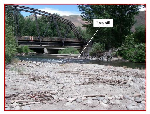
Figure 59. Photograph looking downstream at point bar enlargement, installed rock sill, and bridges in the Highway 75 Reach.
