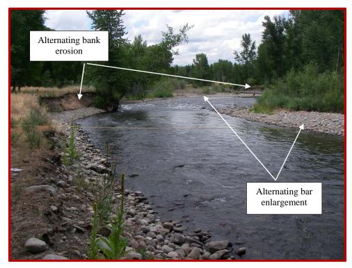
Figure 58. Photograph looking upstream at typical conditions in the Highway 75 Reach.
