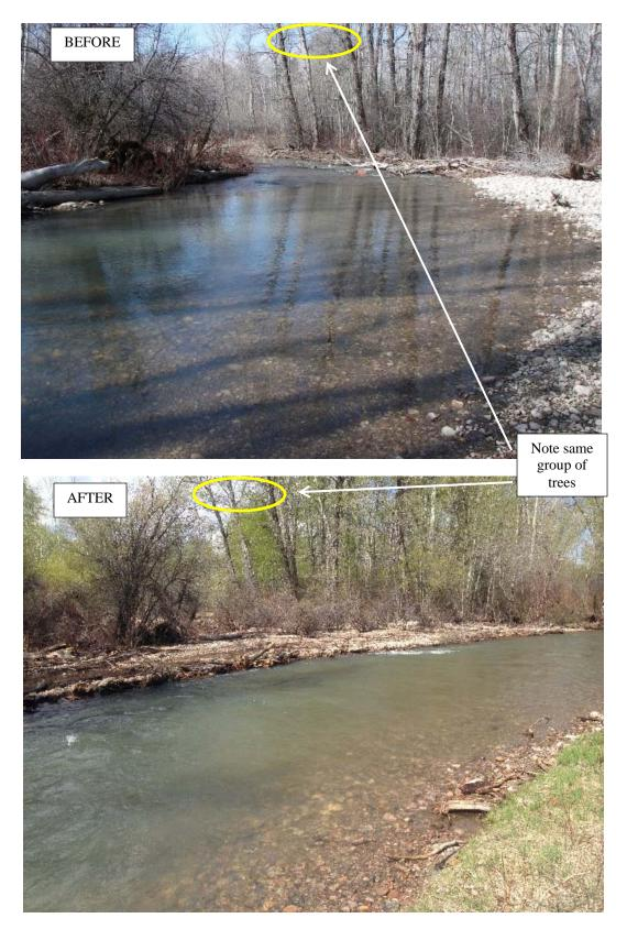
Figure 125. Floodplain creation was used to fill a braided channel network and restore functional channel width within a re-activated historic channel alignment. The treatment achieved flood water dissipation across the floodplain, increased riparian vegetation complexity and abundance, and improved fish habitat associated with increased depth, turbulence, and structural cover.
