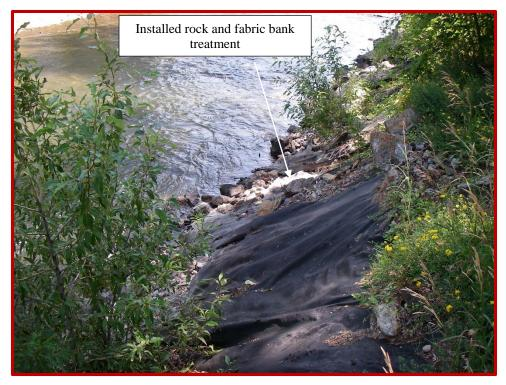
Figure 96. Photograph of installed bank stabilization treatment in the Broadford Street Bridge Reach.
