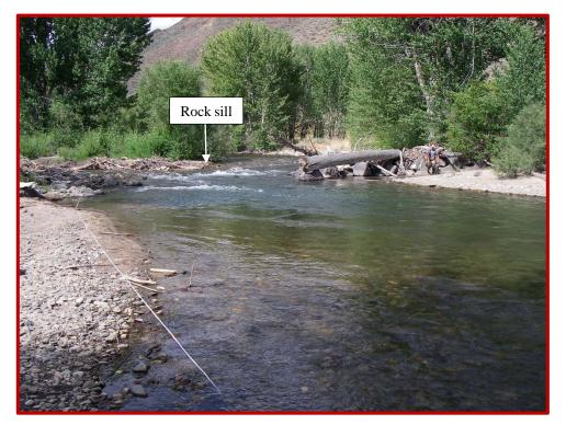
Figure 40. Photograph looking upstream at constructed rock sill, depositional side bars, and confluence of split channel configuration in Hulen Meadows Reach.
