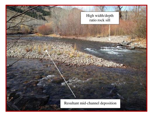
Figure 29. Photograph depicting an installed rock sill and resultant sedimentation in the Training Channel Reach.
