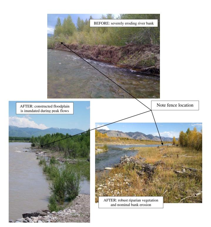
Figure 124. A floodplain bench was created within an over-widened reach of river to eliminate severe bank erosion (top), promote over-land flooding (bottom left), and aquatic conditions and riparian vegetation (bottom right).
